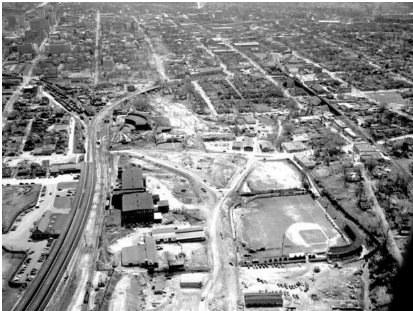
New construction of Capitol Blvd.
